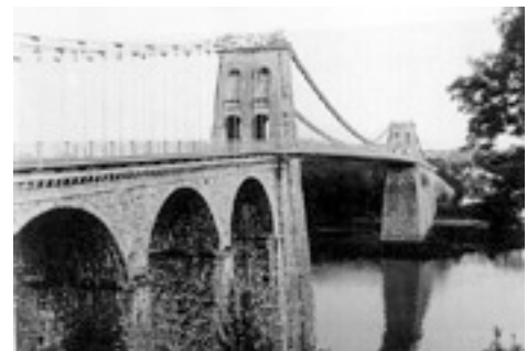
The MENAI BRIDGE, out to Anglesey, designed by Thomas Telford and built in 1826
